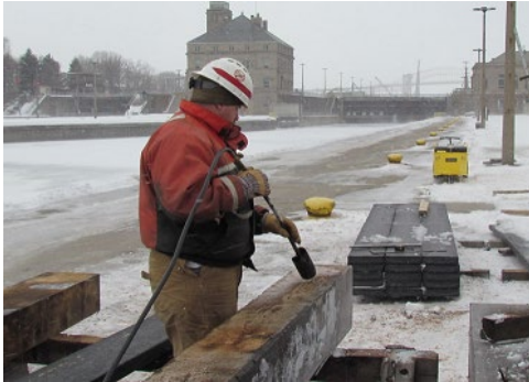
Image courtesy USACE Sault Sainte Marie, Ice Fender Repair at Soo Locks
