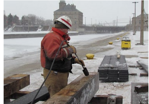
Image courtesy USACE Sault Sainte Marie, Ice Fender Repair at Soo Locks
