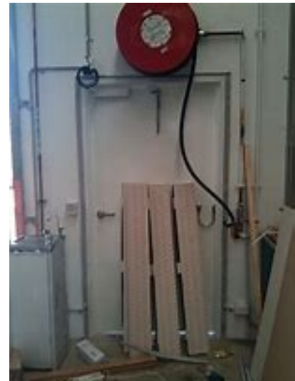
Picture shows a blocked and unmarked exit Image retrieved from Bing Images (free to share and use license)
